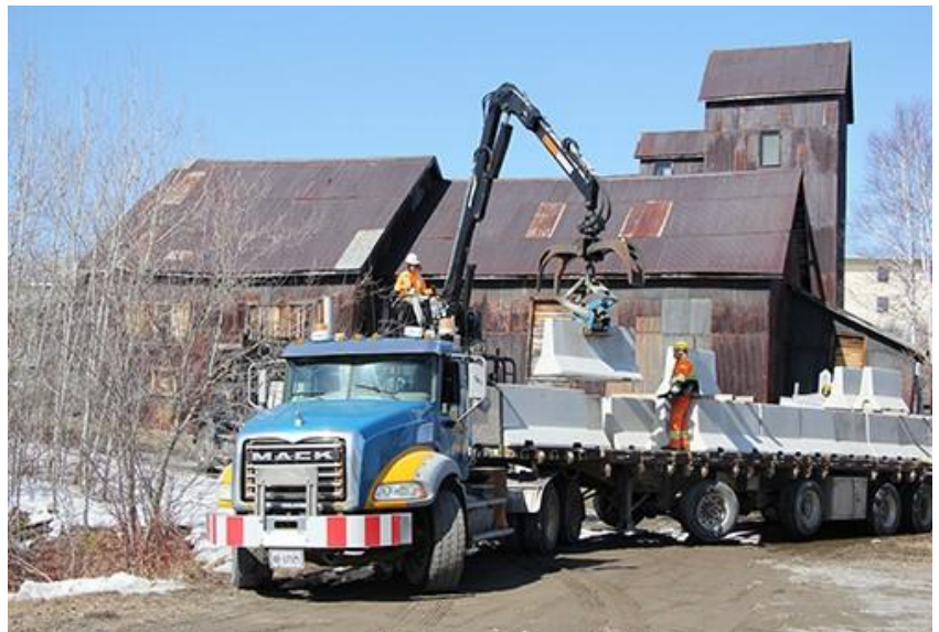
O.N..R placing concrete barriers at the Right of Way Minesite in March 2021.
