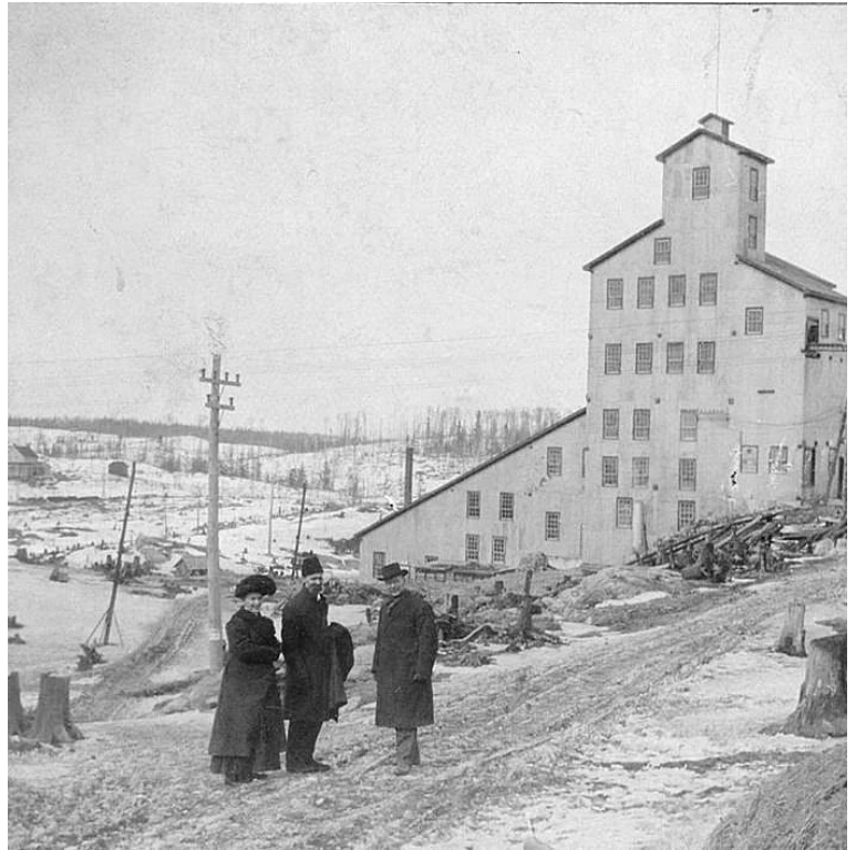
In 1910, visitors could easily walk to the Trethewey Mill near Sass Lake. Today, the site is completely overgrown.
