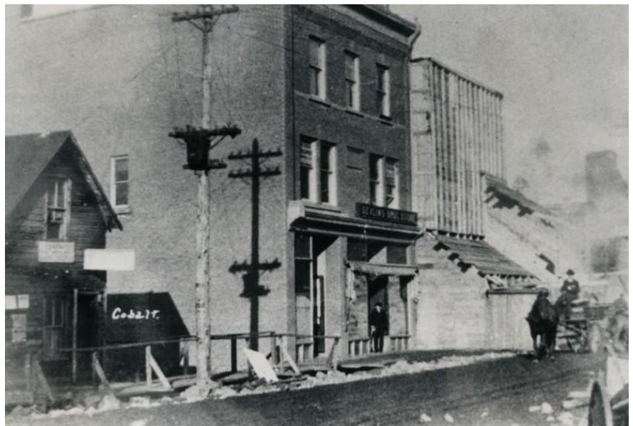
Devlin Block next to the Royal Exchange Building aka Bilsky Block under construction ca 1909.
