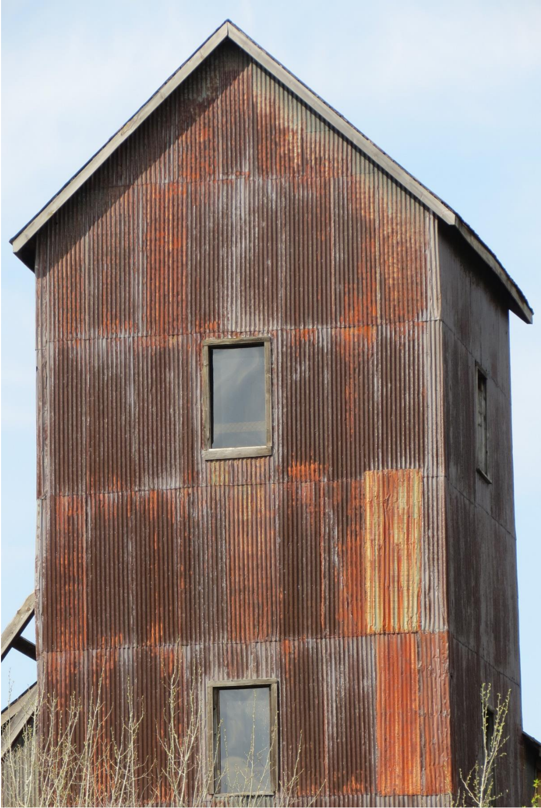
Right of Way Mine – No. 2 shaft (exterior cladding)
