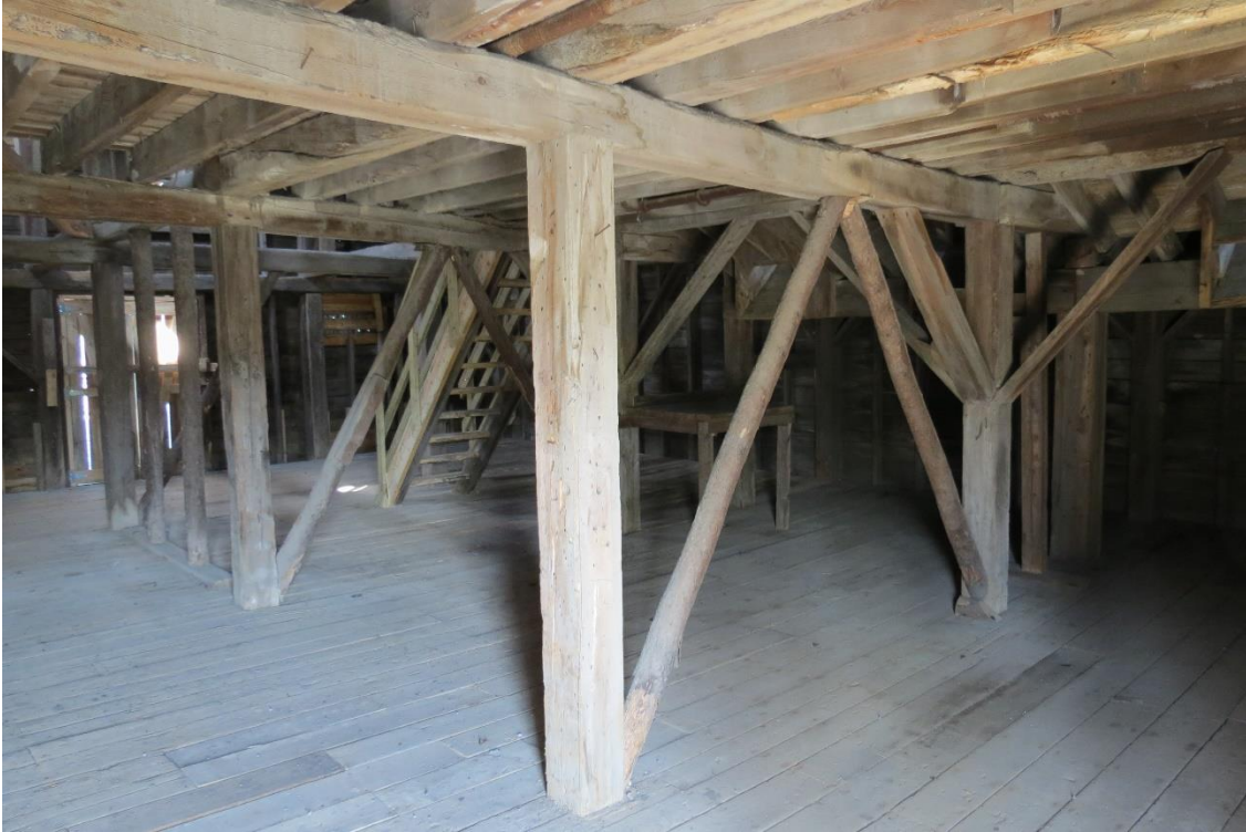
Right of Way mine – No. 2 shaft interior timbering
