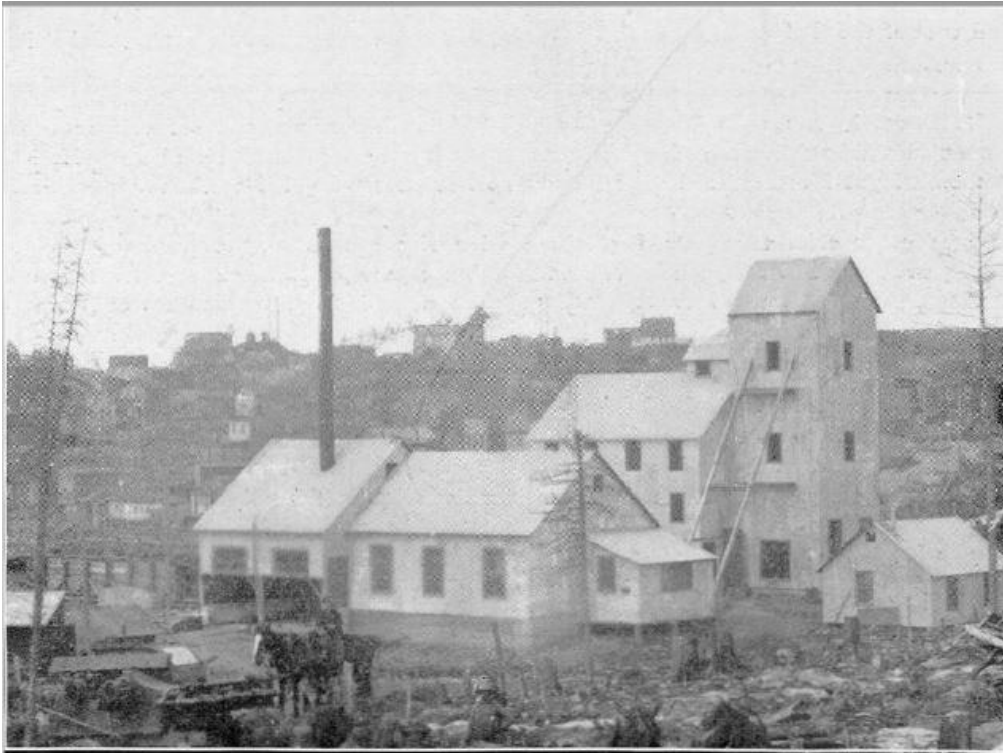
Right of Way Mining Company – No. 2 shaft looking westerly. Ontario Bureau of Mines
