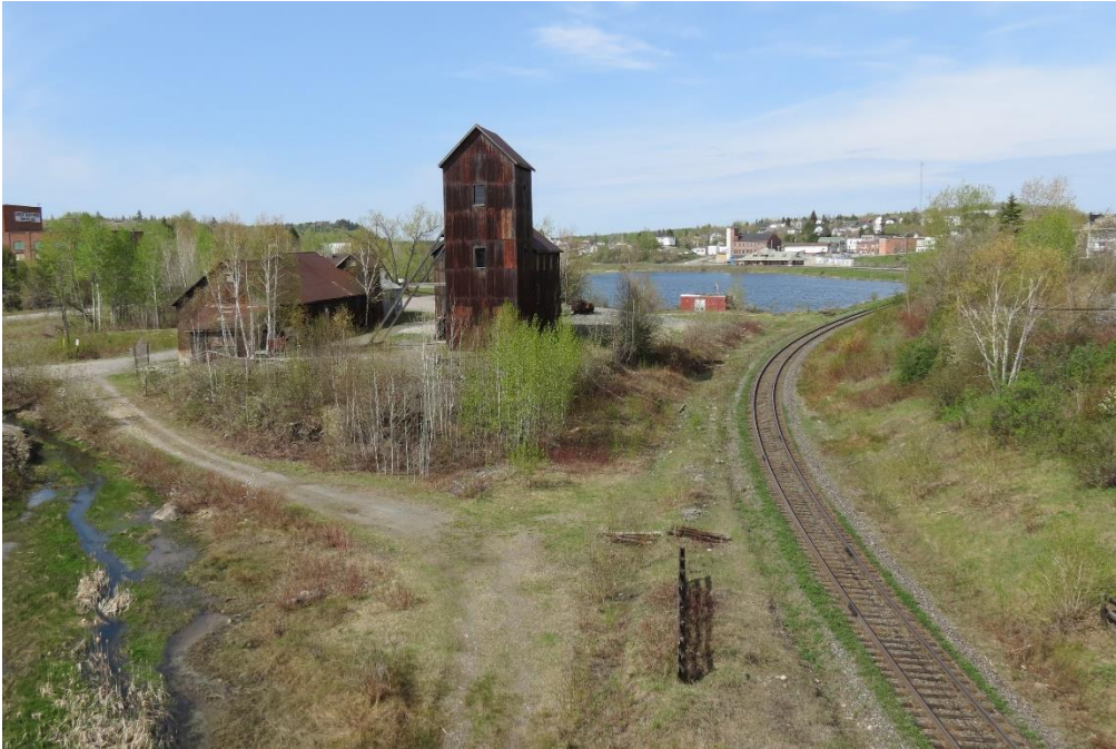
Right of Way mine – No. 2 shaft (looking south toward Cobalt Lake Allan Stacey©
