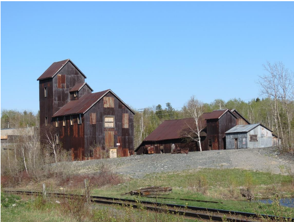
Right of Way mine - No. 2 shaft (looking northeast)
