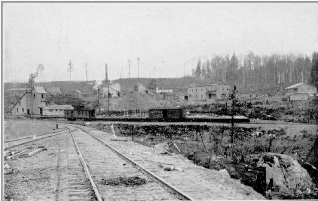
Right of Way Mining Company – No. 3 shaft extreme left – looking southwesterly. The Silver Queen Mine is just to the right and is the white structure. Ontario Bureau of Mines
