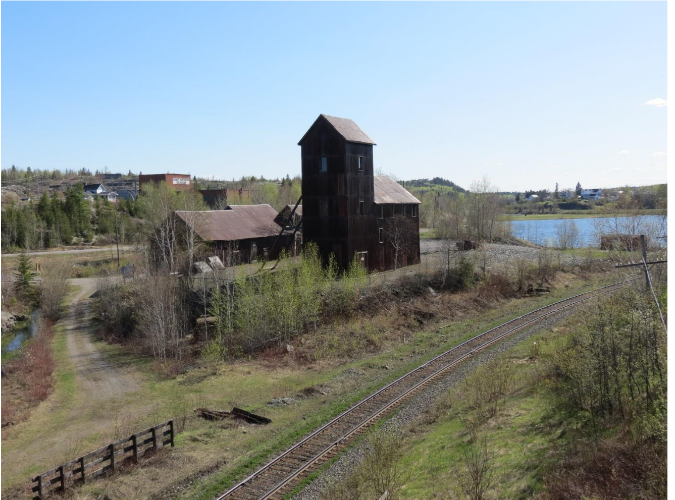
Right of Way Mine – No. 2 shaft looking southerly to Cobalt Lake
