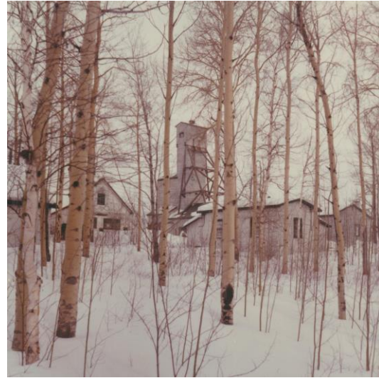
O'Brien mine of Agnico Mines, Limited in winter 1970. The author began hard rock mining at this location in 1965. - Author's collection ©
