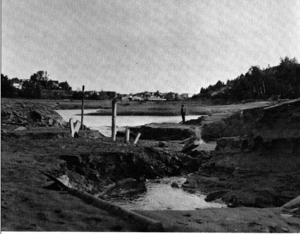
Approximately one million tons of tailings are contained in the bed of Cobalt Lake, containing an estimated average of four ounces of silver per ton.
