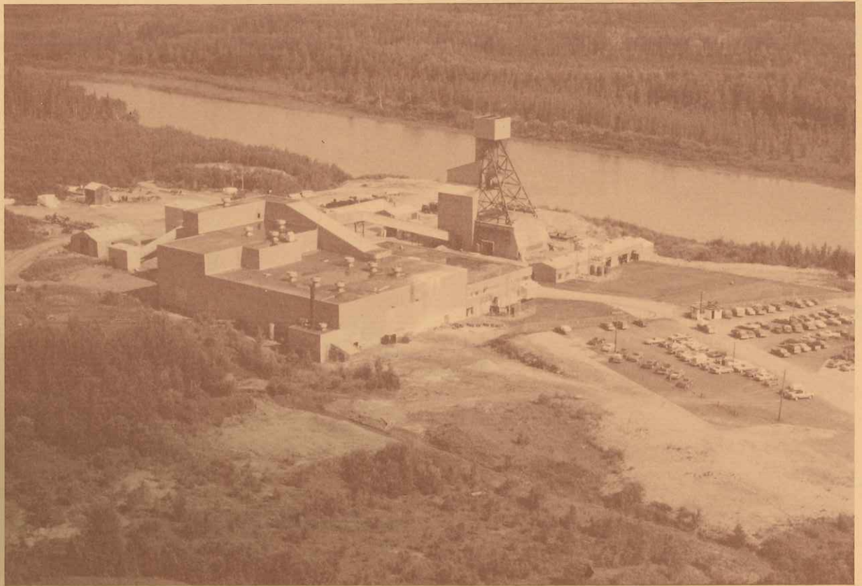
Today the Eagle mining, milling and refining complex supports a staff of over 280 employees
