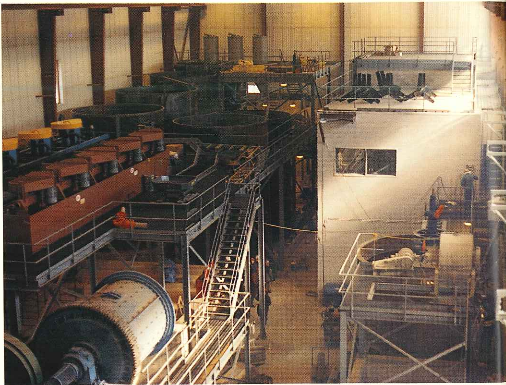
The mill interior, showing the carbon-in-pulp and flotation areas. Photograph was taken March 11, 1988
