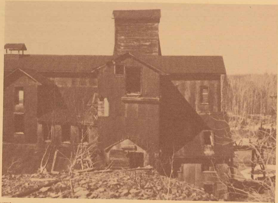
"The rusting skeletons of abandoned headframes"
