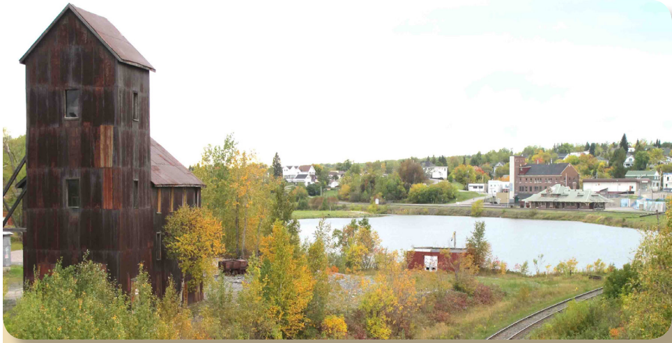
The Right-of-Way Mine headframe rises above the shores of Cobalt Lake on the outskirts of Cobalt.
