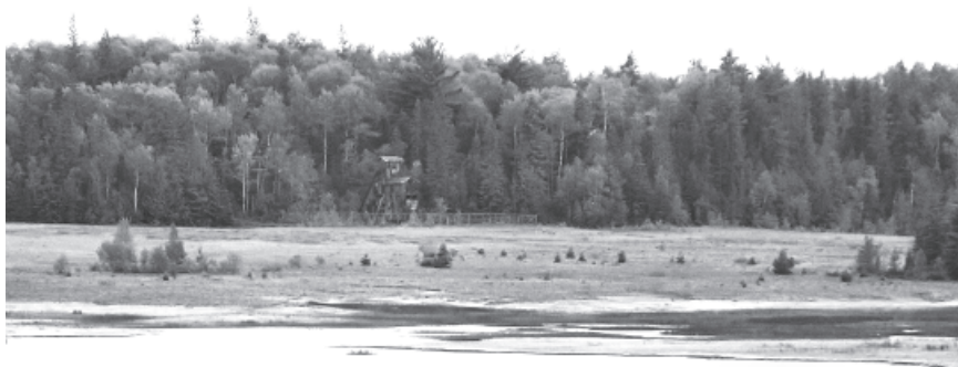
Across Cart Lake, Provincial head frame fenced off for safety reasons.
