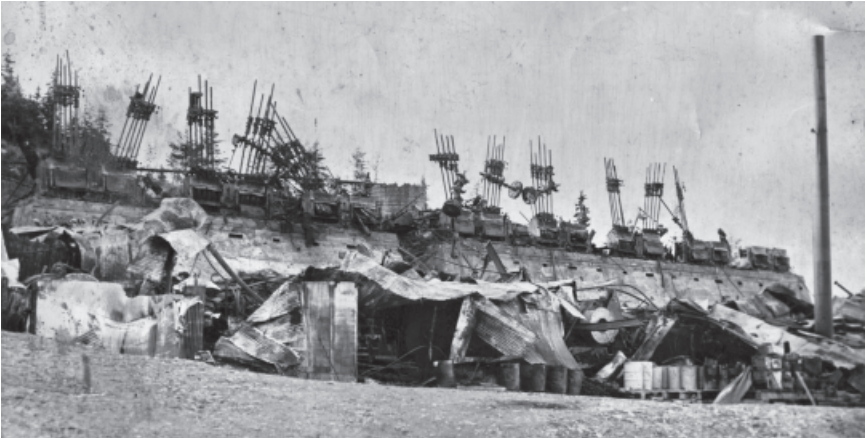
104 Mill after the 1956 fire revealing the remains of the stamps.
