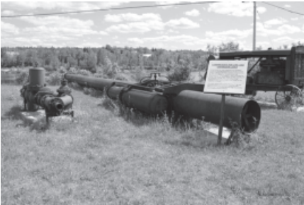
Expansion Joint from the Ragged Chutes Air Plant system
